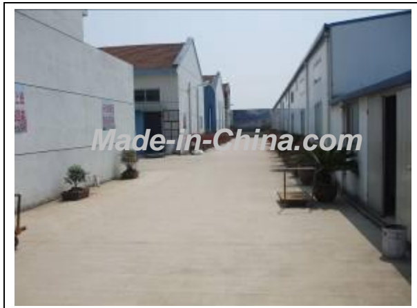
Description: Workshop building
